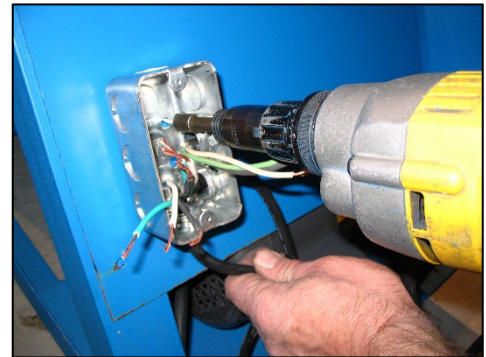
Step 9: Connect wires per schematic. Connect all three ground wires and attach mechanically to box per code. Wire nut all connections.
