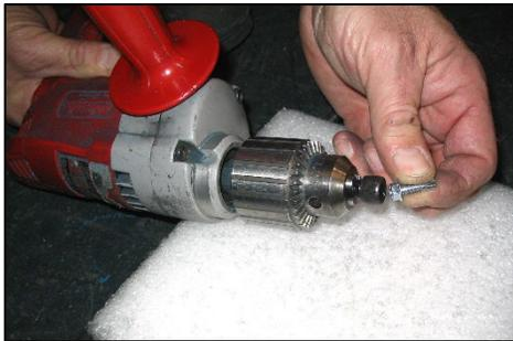
Step 2: Use a drill to remove the self drilling screws from the cover, by inserting the provided bolt to act as a 5/16" screw socket.
