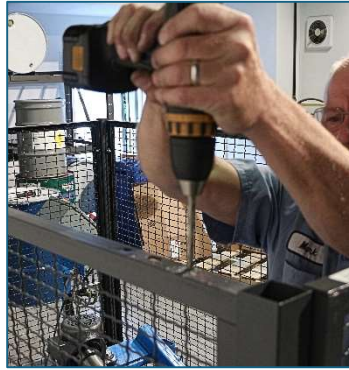
Drill holes for switch mounting plate.
