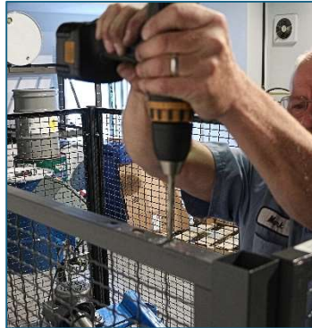
Drill holes for switch mounting plate.
