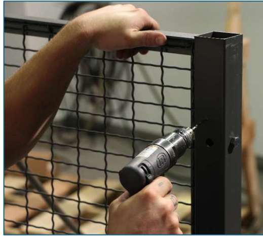
Drill holes for hinges in posts to mount door at desired height.
