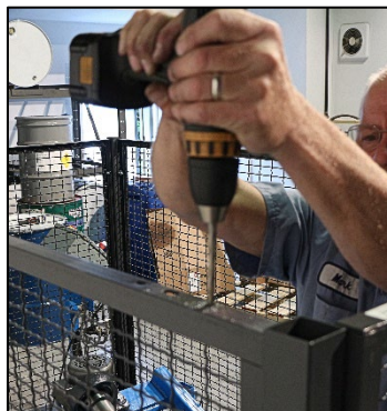
Drill holes for switch mounting plate.
