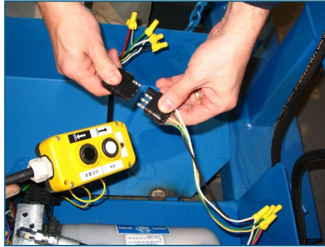
12. For pendant operation, plug male plug from pendant into female plug of pump.
