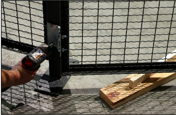
Attach bottom door hinge to post with self-tapping screws.
