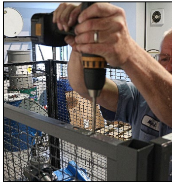
Drill holes for switch mounting plate.
