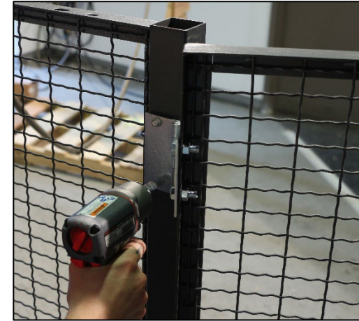
Attach top door hinge to post with self-tapping screws.
